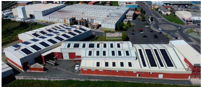
INTAF GROUP S.A. 329.85 KWp photovoltaic self-consumption plant in A Coruña, Galicia. Finished in February
