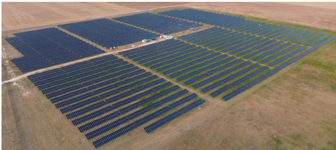
Villanubla Solar 10.39MW photovoltaic generation park in Castilla y León, Valladolid.
